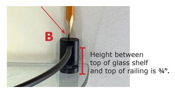
3. Using a level, confirm the horizontal position of each *screw location*.
