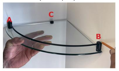
2. Mark the wall surface with a **vertical pencil mark** at the **centre** of each wall flange.
